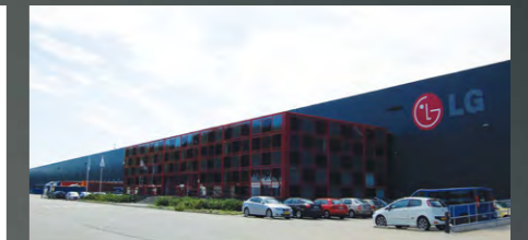
European Air Conditioning Distribution Center
