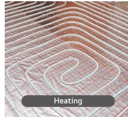
Radiant Heating / Cooling
