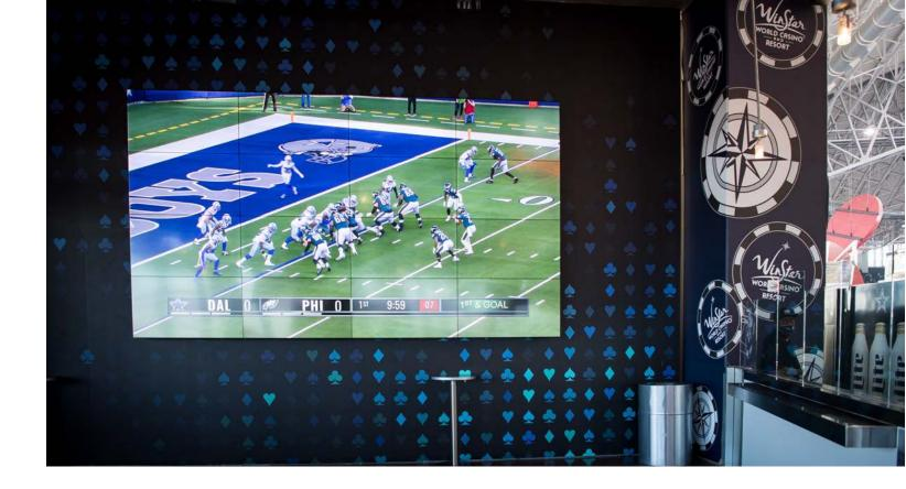
For even greater impact, several areas now feature large scale video walls comprising multiple LG displays, including a 5x5 wall in an upper concourse bar that uses 25 55-inch displays, and walkway areas with three 75-inch displays mounted vertically sideby-side to use as a video wall or as three separate displays.
